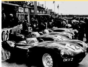
technology produced a very slippery car. The XK based engine powered the D type. It now produced 245 bhp thanks to a revised block, larger valves and the triple Webber carburettors. It now had the potential to top 170 mph.
